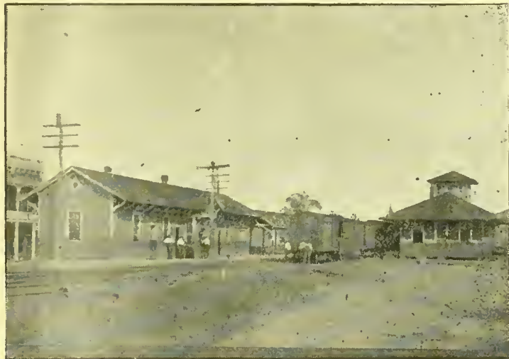
Passenger and Freight Depot of Southern Railway
